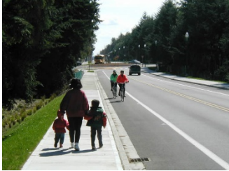
Complete streets are thoroughfares that are planned, designed and constructed to allow access to all legal users safely and efficiently, without any one user taking priority over another.
